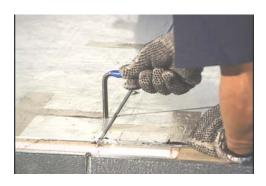
5. Check to see if F8A and F8C floor panels are firmly attached together. If not, repeat this step. If tight, lock remaining cams and go to the next panel until all floor panels are assembled
