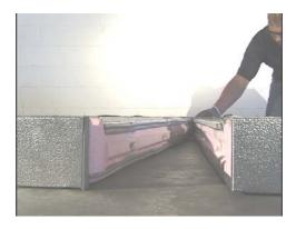
4. Insert cam wrench into center hole on panel F8A. Turn wrench in clockwise direction until stop is felt. (See Cam description)
