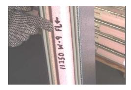
4. Once these two panels are in place and are flush at the top with each other and flush at the bottom with the floor panels, take the cam wrench and insert into the center hold of the W1 panel.
