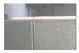
7. Lock the door before installing the door panel. Set the panel in place. The perimeter of the door should be flush before locking it in place.
