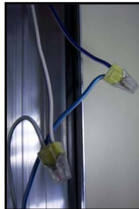
3.5 If no connector is found on driver, cut off power wires from frame harness as shown and connect wires together using Wago connector Part# 773-162 or other approved connector.
