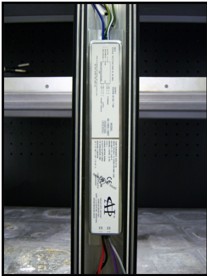
3.1 Install Driver in the same location where the ballast was fitted using existing self-tapping screws. (Driver may have to be moved up or down to coincide with hole pattern)
