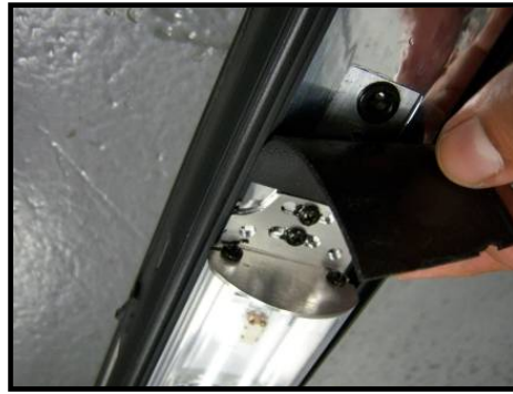
2.5 Cover exposed holes using supplied seal foam tape as shown (top of light fixture).
