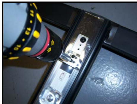
2.8 Using fixture as a template, drill two Ø.106 (#36) holes through center and end mullions making sure wires inside mullions don't get damaged.
