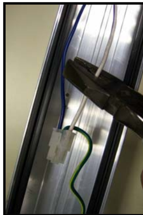
3.5 If no connector is found on driver, cut off power wires from frame harness as shown and connect wires together using Wago connector Part# 773-162 or other approved connector.
