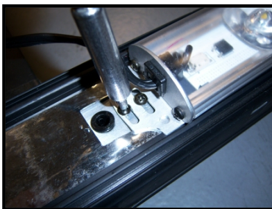
2.7 Place LED fixture on mullion making sure that slots line up with existing bottom holes in the frame and attach it using screws as seen on step 2.4.
