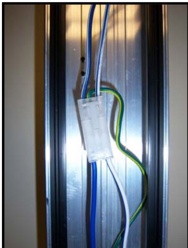
3.4 Connect driver's input wires (Blue and White) to power harness from frame as shown.
