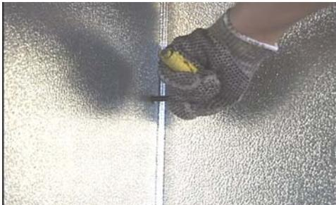
5. Turn wrench in a clockwise direction until stop is felt. (See Cam Lock description) Check to see if panels are firmly locked together. If not, repeat this step.
