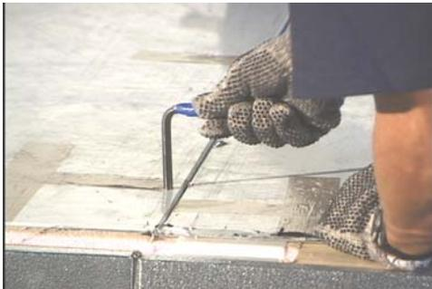
5. Check to see if F8A and F8C floor panels are firmly attached together. If not, repeat this step. If tight, lock remaining cams and go to the next panel until all floor panels are assembled
